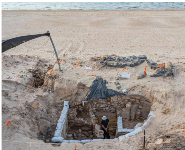
Figure 28. Eastward oblique view of the excavated (in 2021) structure on a western berm demonstrating the depth of the foundations or multi-stage remains solely containing Early Islamic-dominated artifacts.
